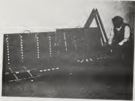
Figure 5. Mockup during assembly.
